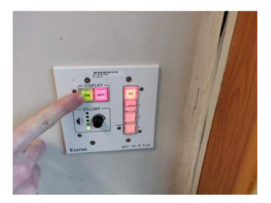
To adjust the volume on when using the HDMI audio input, turn the knob labelled 'volume' on the wall panel.
